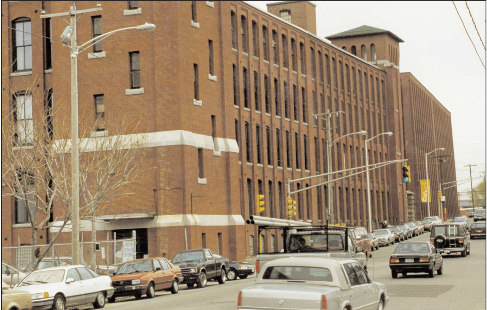
12. An idea of the scale of the combustible mill buildings that were involved in this incident.
