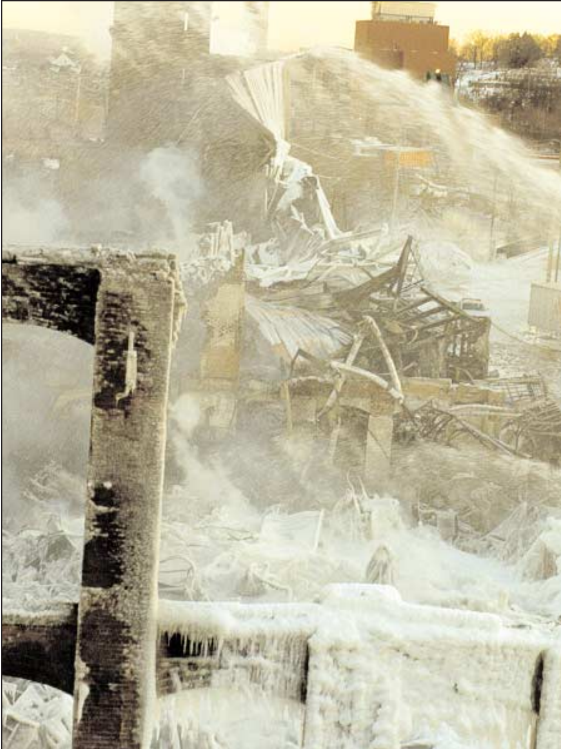
5. Remains of the Monomac Building looking to the south.
