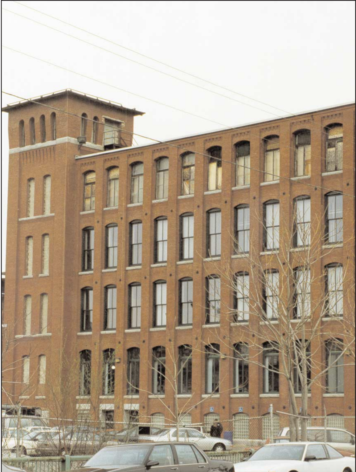
10. Example of the heavy masonry buildings that were involved in the fire.
