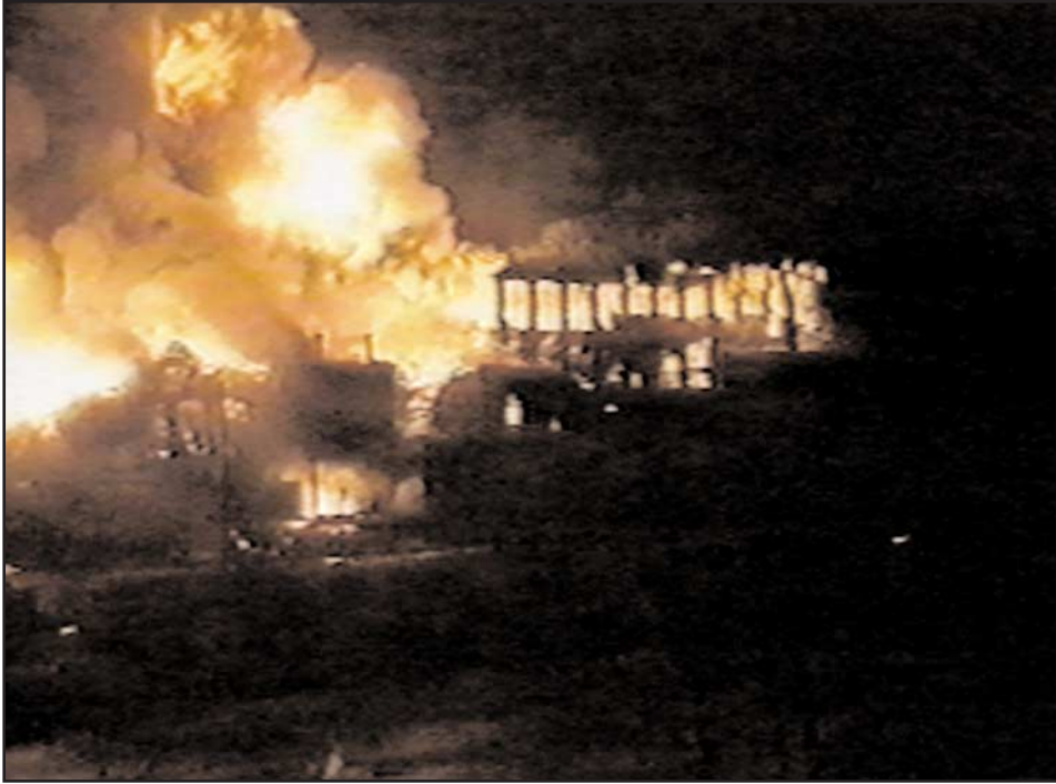
2. The fully involved west side of the Monomac Building; floors have collapsed as have some walls. Vantage point was across the Spickett River.
